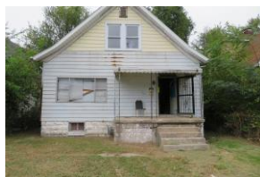
443 North 22 nd Street, ESL 2-bedroom home, basement
