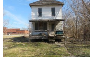
1506 North 41 st Street, ESL – Large 3-bedroom home, basement
