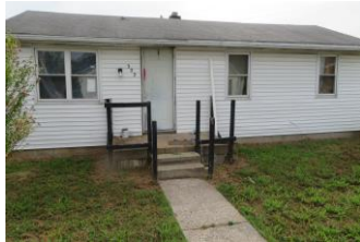
509 South 5 th St. LVJ $29,900 $900 Down/$500 a Month
