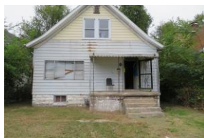
443 North 22 nd Street, ESL 2-bedroom home, basement
