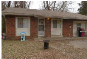
2304 North 60 th Street, WP Brick 3-Bedroom home
