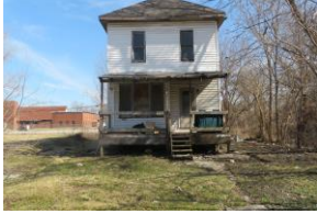
1506 North 41 st Street, ESL Large 3-bedroom home, basement
