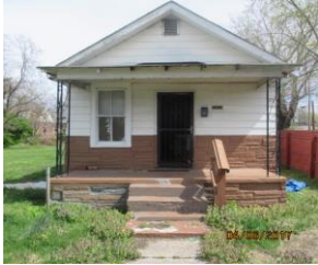
2433 St. Louis Ave. COMING SOON!!
